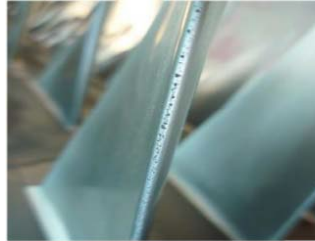
Corrosion Pits on the Leading Edge of Compressor
